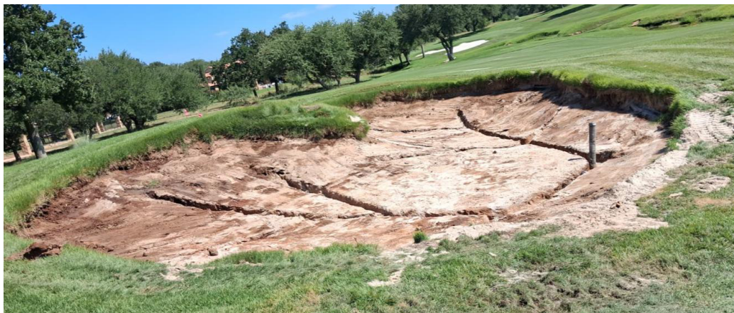
Fairway Bunker, Hole #16: Existing Sand, Drainage and Liner Removed
