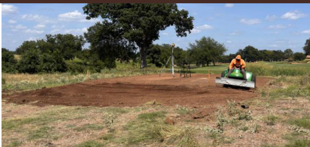
Hole #18: New Tee Complex Under Construction
