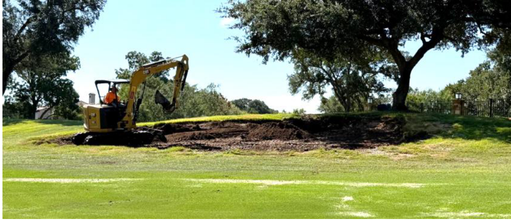
Fairway Bunker, Hole #18: Bunker Eliminated and Filled With Soil
