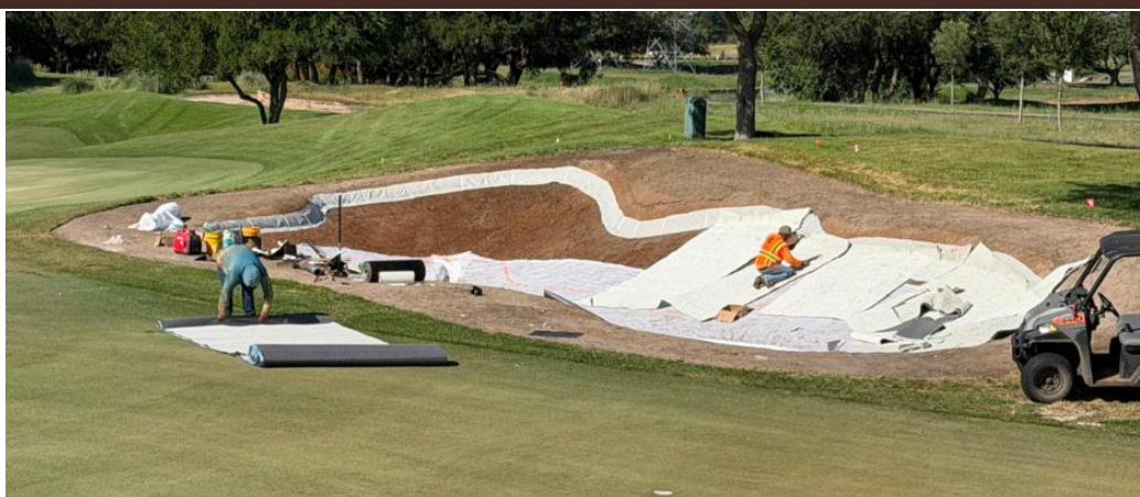
Fairway Bunker, Hole #11: Bunker Solution Liner Installed
